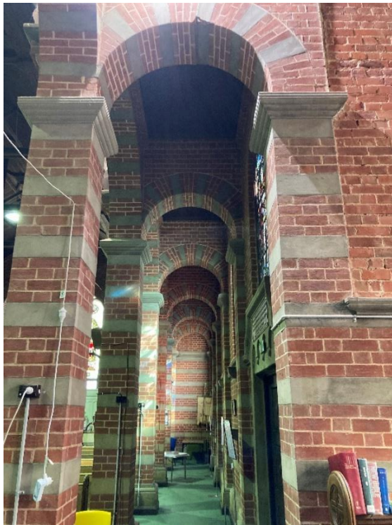
Arcades featuring Tuscan columns with round-headed arches, featuring polychrome work with alternating bands of cement and red face-brick to voussoirs and columns, form the aisles of the church.
