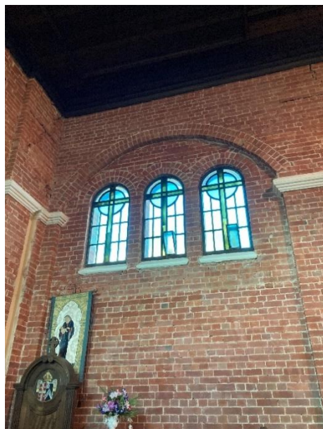
Lead light in the triplet windows. Note the poorer condition of the brick face due to the removal of the plaster from this part of the church.
