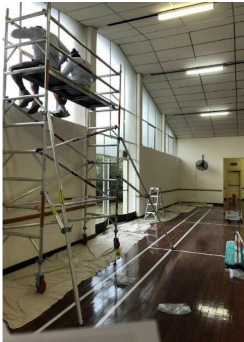
Coles Hall repainting underway
